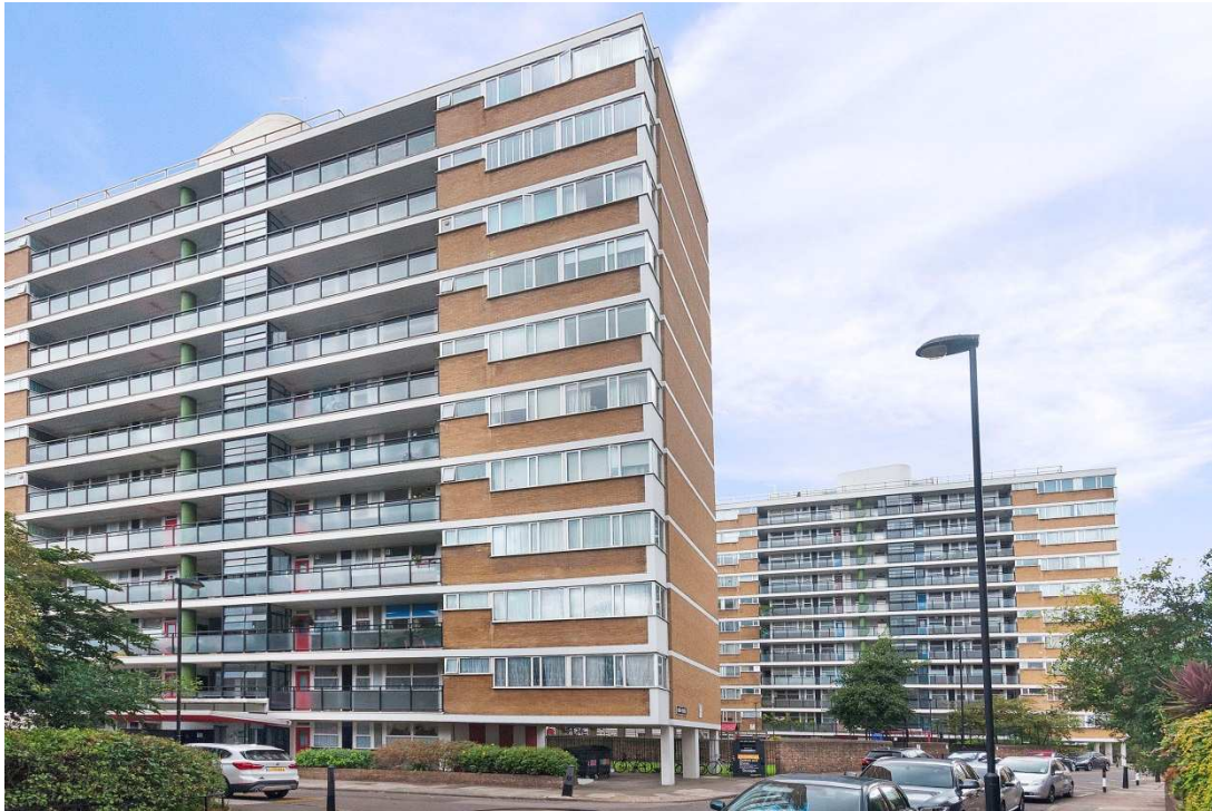
Sheraton, Ripley and Anson, Churchill Gardens estate, 11 storeys
